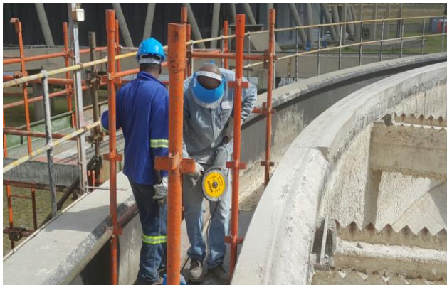
Repair of damaged concrete on a clarifier at Eskom Lethabo Power Station
