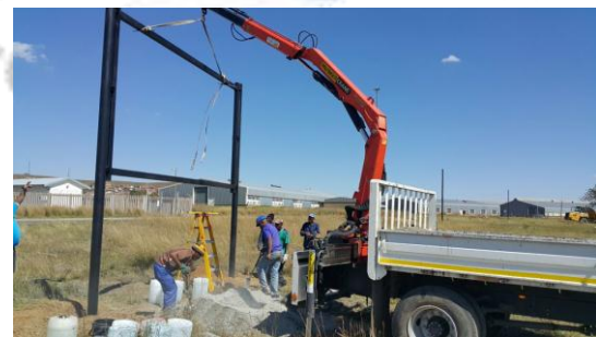
Erecting the Bill Board Frames in Harrismith for FDC.
