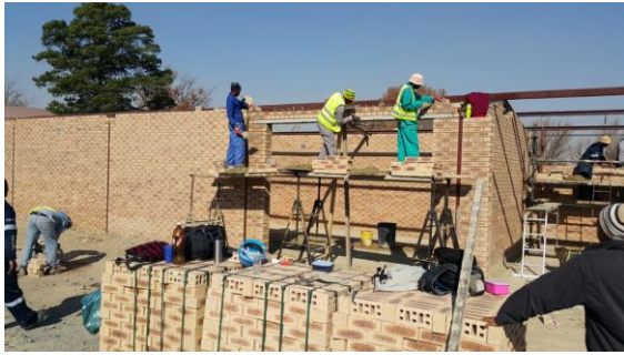
Bricklaying is almost complete on a 3m high warehouse.
