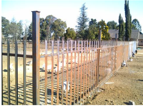
Erection of pallisade fencing at a private house in De Deur.
