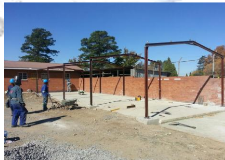
IPE Sections are erected before the laying of the bricks.
