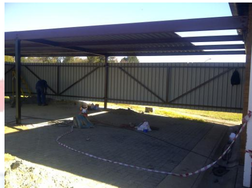
Fabrication and Erection of a carport at Rand Water.
