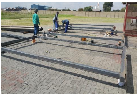
Manufacturing of Steel Bill Board Frames for Free State Development Corporation
