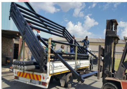
Loading and transporting the steel frames to Site.
